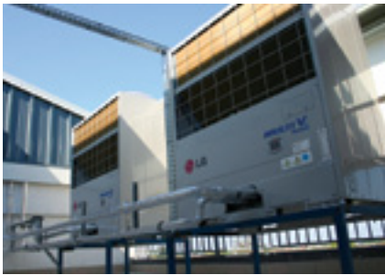
The school built a new gym and the cooling and heating system is provided by LG Multi V. It cools down and heats the entire sport hall, the connected areas, and dressing rooms.
